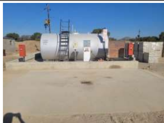
Photo 4-2 Spill slab at refuelling point
