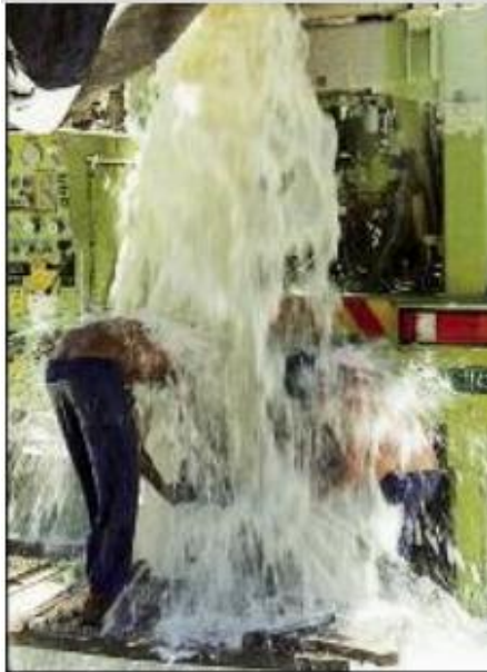
Under pressure! Borehole penetrating the Oshivelo Artesian Aquifer with a free flowing yield of more than 200 m 3 /h.
