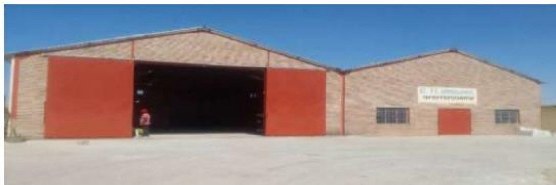
Figure 3: Existing BH Spares warehousing
