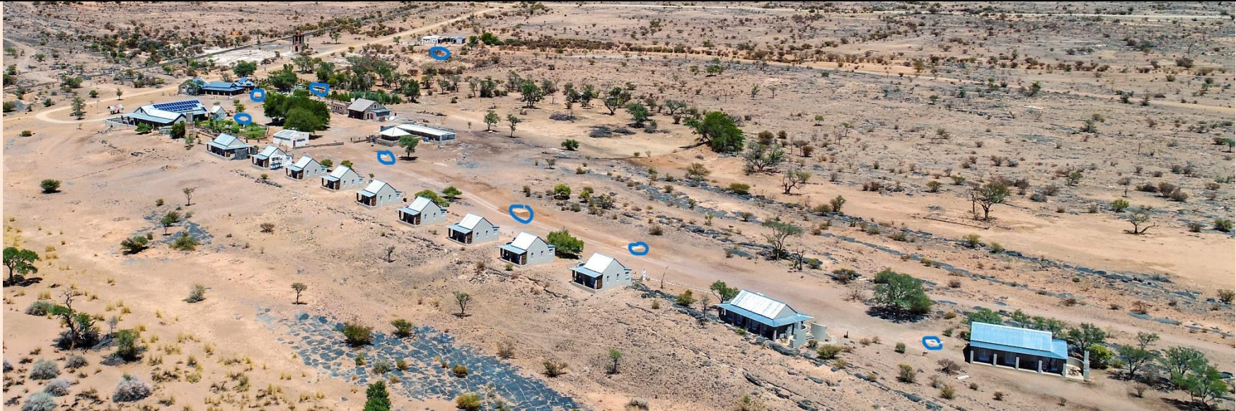
Figure 5: Picture showing the location (blue circles) of the eight, two-chamber French drains (Source: Mr Frikkie Mouton, Manager, Alte Kalköfen Lodge).
